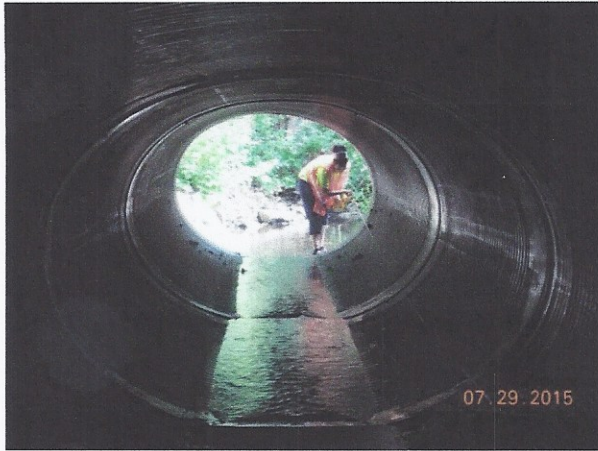
Fern Mastroluca taking field measurements of a corrugated road culvert
