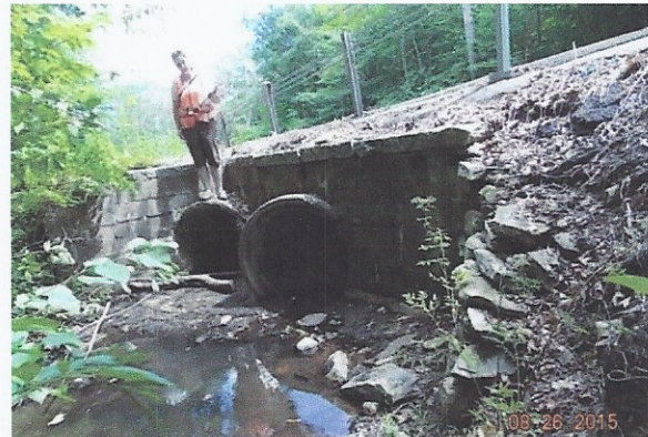
Bobbi DesRoche evaluating passage barriers at culvert inlet
